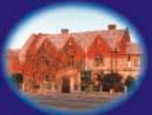
The Hotel at Hopcrofts Holt
